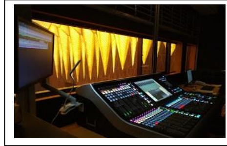
Ruang Kontrol (FOH)
